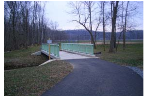
Phase 1A Bridge on Pleasureville Boys Club Crist Fields
